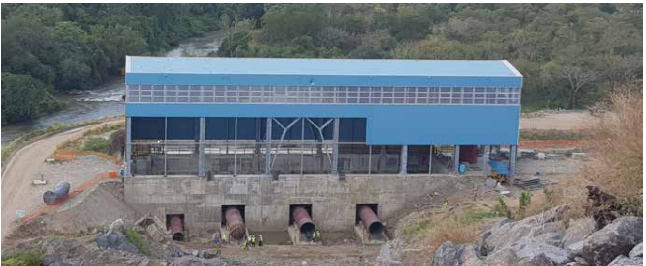
The power house in which the turbine exhaust pipes will be installed.
