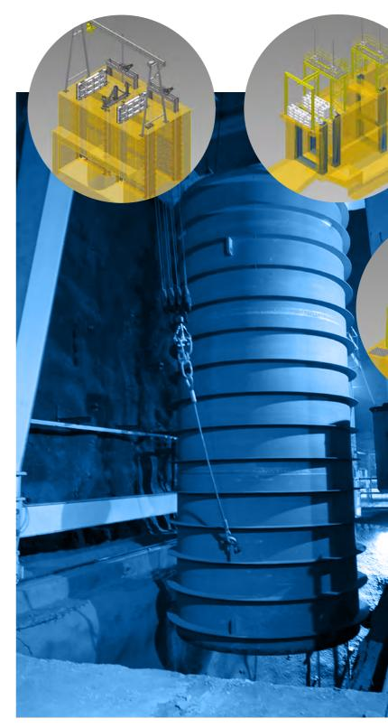
↑ Alto Maipo Hydroelectric Project (Chile) N.2 Penstocks: ID 3,700 mm and 2,400 mm Vertical shaft 551m depth Material EN10025-6 S690QL
